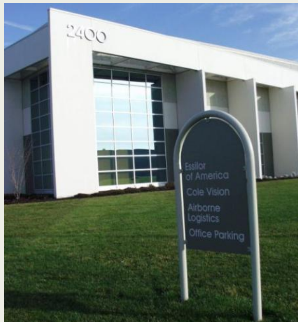
Well-designed industrial development.
